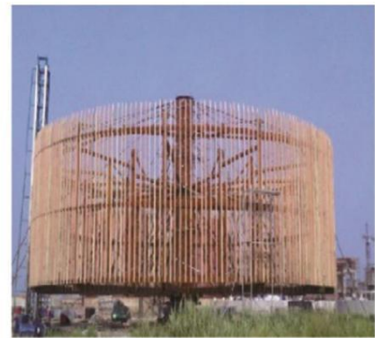
现场缠绕设备 Field winding equipment
